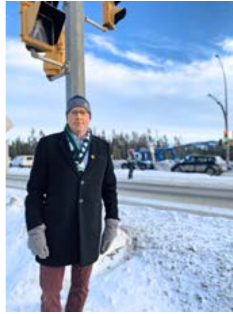
Minister of Highways and Public Works Nils Clarke checks out the new advanced left turn light being installed at the Robert Service Way and Alaska Highway intersection in Whitehorse.
